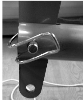
Join the leg section tube with the leg section bracket, using a pipe pin in the upper hole of the bracket.
